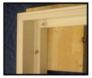
6. Position the assembled frame evenly around the window opening & secure with nail/screw (pre-drill) into the upper left frame <u>ONLY</u>. Shutter will be fully secured in later steps.
