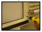
Only secure <u>one</u> screw into the bottom right frame.
