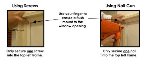
Tip: It is best to angle the drill gun or nail gun to ensure contact with a stud around the window opening.
