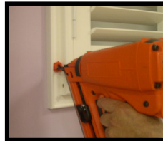
Only secure one nail into the bottom left frame.
