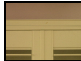
Double Check panels before securing.
