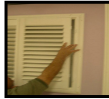
Insert panel into position.
