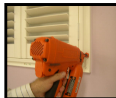
Only secure one nail into the bottom right frame.
