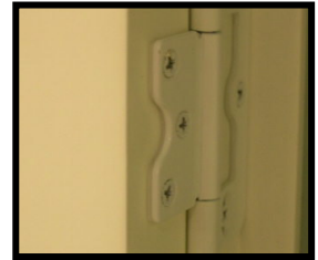
Hinge spacer installed
