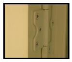
Hinge spacer installed
