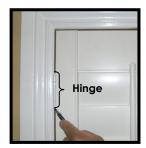
Mark should be made on the wall/jam at the bottom of the hinge.
