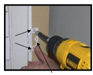
Note: If the panel has more than 2 hinges, go ahead and install the screws to the rest of the hinges.
